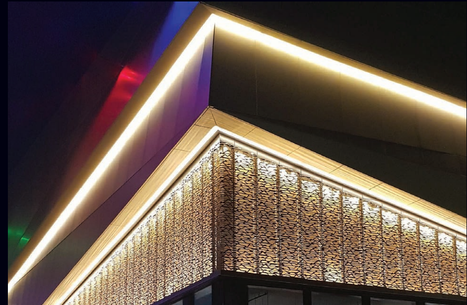
Intu Lakeside Shopping Centre. Lighting design by Hoare Lea
