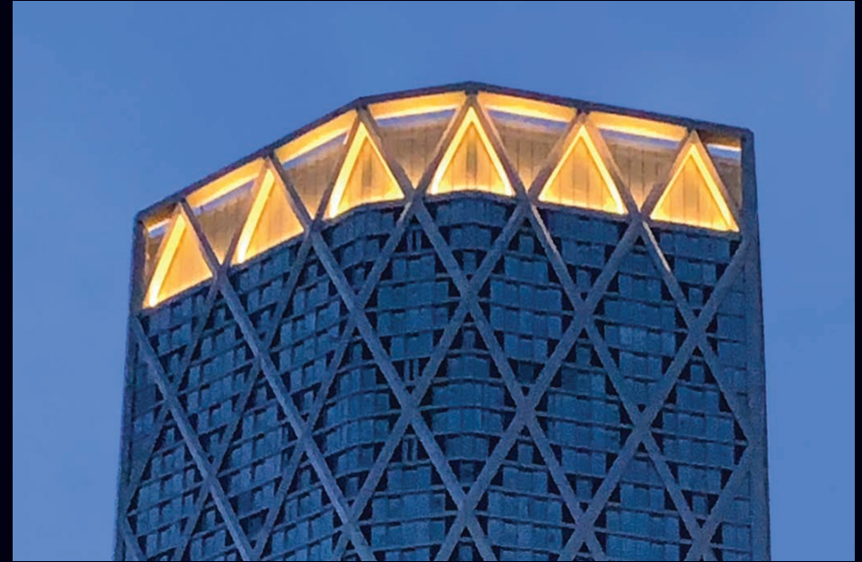
Newfoundland Tower, London. Lighting design by MBLD
