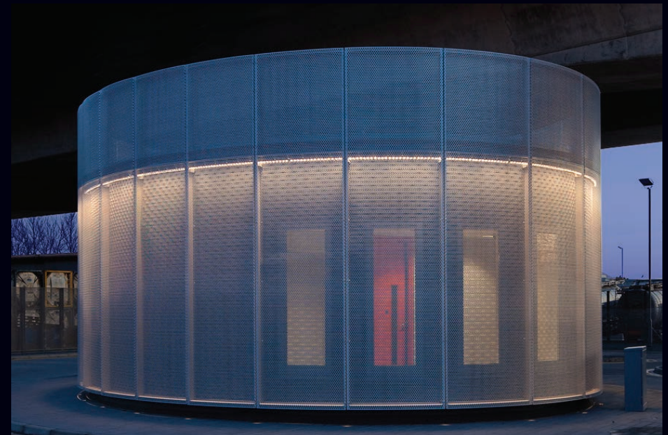
TFL project. Architect Burns and Nice. RIBA award winner
