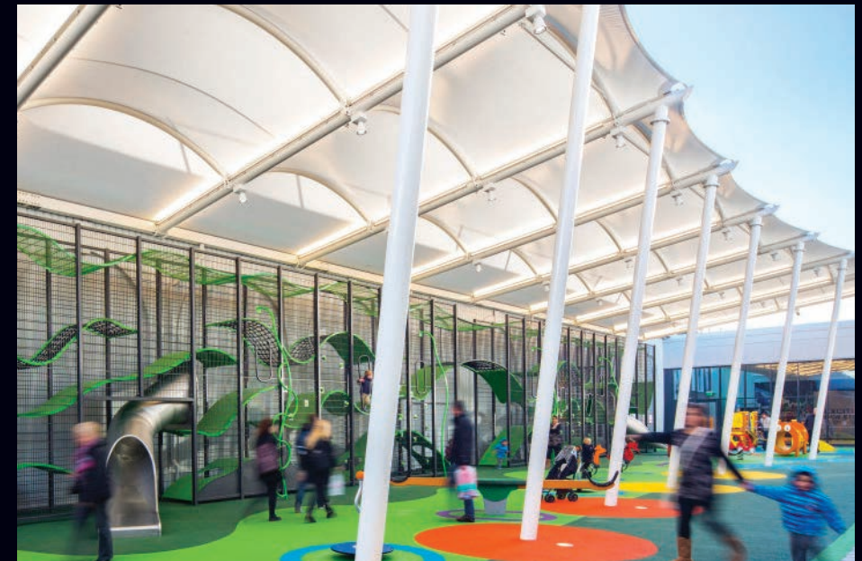
Swindon Designer Outlet, UK. Architecture by McLaren & POD. Lighting design by Aecom
